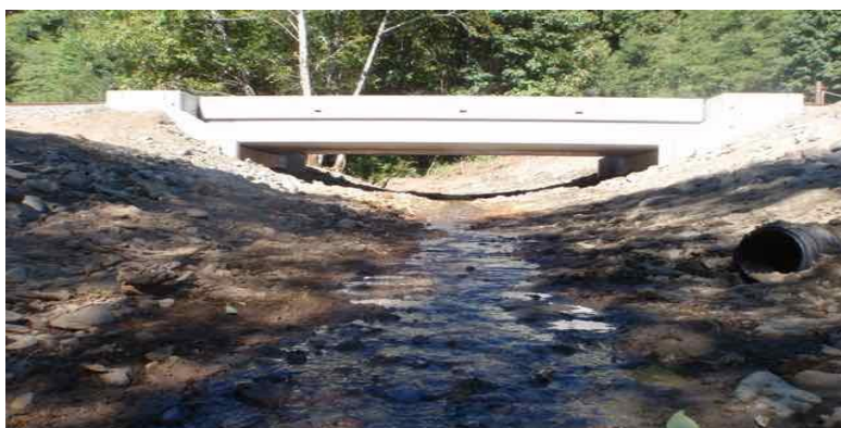
Figure 6: Completed culvert Project
