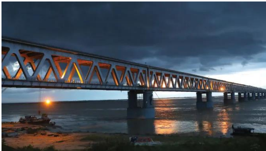
Figure 2: Bogibel Bridge in Assam (Source: India Infrastructure)
