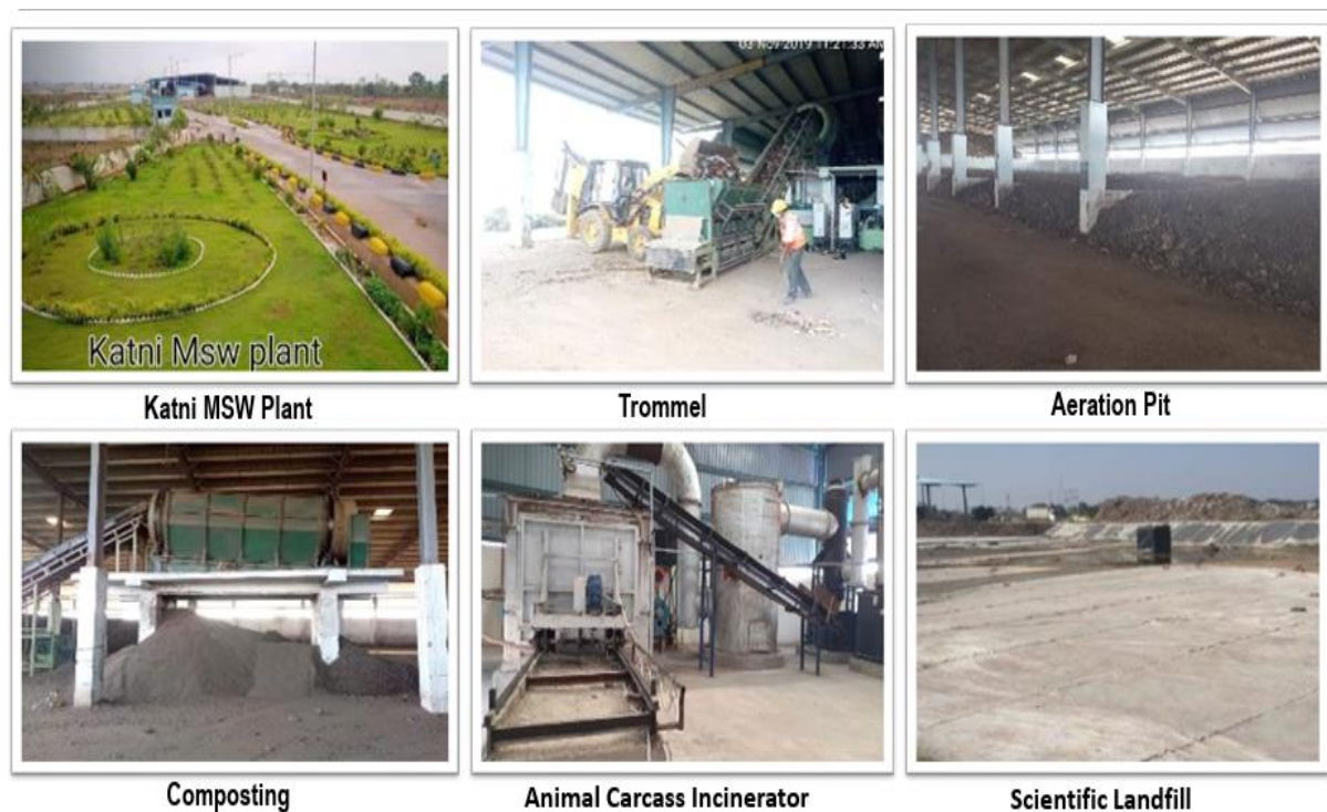
Figure 22 Waste Processing Plant & Scientific Landfill of Integrated Solid Waste Management, Kanti cluster
