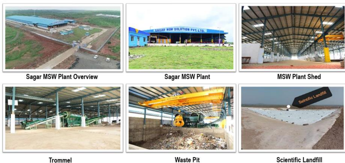
Figure 23 Waste Processing Plant & Scientific Landfill photos of Integrated Solid Waste Management, Sagar cluster
